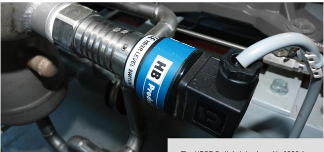
The mechanical section of the HBSR switch has no moving parts and a lifespan that can be longer than the refrigeration system itself. However, the electronic part of any switch is more fragile and can become technically obsolete over the years. The split design therefore simplifies the maintenance by allowing easy replacement of only the electronics.
