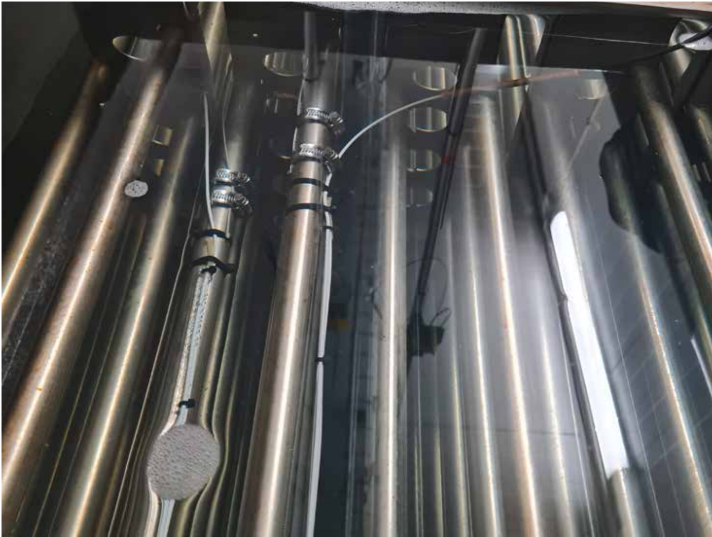
Two Ice Bank Sensors have been installed on the top cooling pipes of an ice bank at a dairy in Sweden. This system is part of an older installation.
