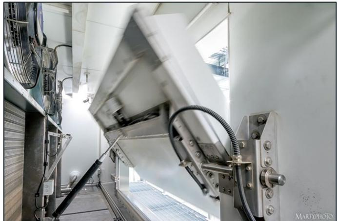
Door for ambient air inlet to evaporator
