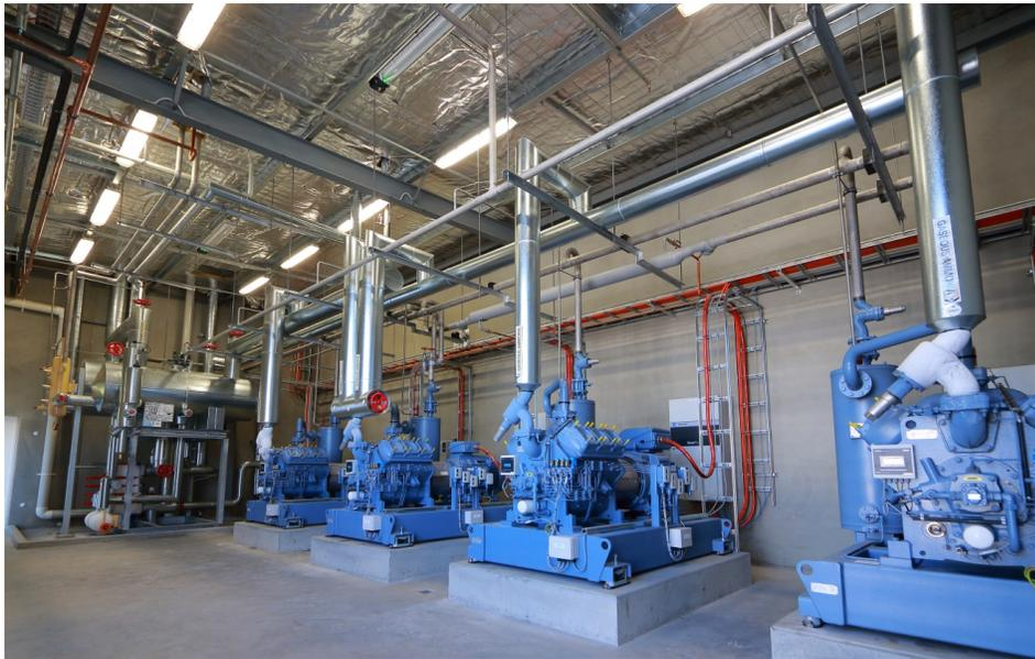
Figure 3. Low charge NH<sub>3</sub> system with secondary refrigerant and energy recovery from the second stage compressor discharge line for the desiccant drier
