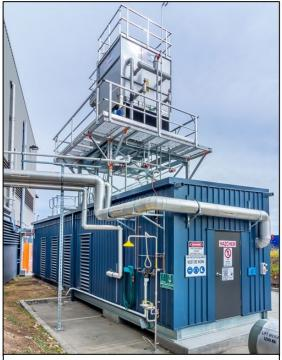
Prefabricated machine room for low charge DX ammonia system
