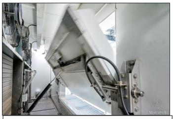
Door for ambient air inlet to evaporator
