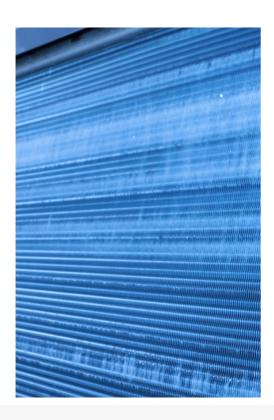
Ice build-up affects the efficiency of the evaporator, therefore it is important to be able to measure the formation of ice and control the defrost in accordance with the conditions.
