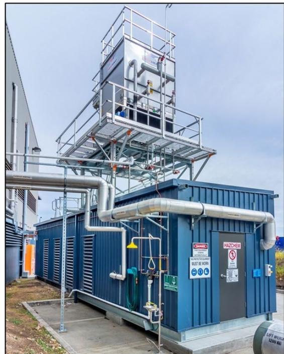
Prefabricated machine room for low charge DX ammonia system
