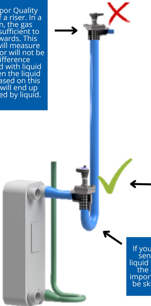
When installed just after the evaporator the sensor can be used to control the liquid feed and secure a riser which is working.
