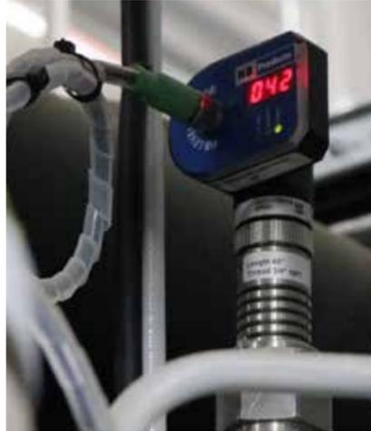
Traditionally DX CO2 systems are controlled by superheat. The superheat calculation is based on a temperature measurement and is a rather slow control system. Vapor Quality Control is an instant measurement system and allows for increased suction pressure and improved COP. A typical energy saving is 15-20 %
